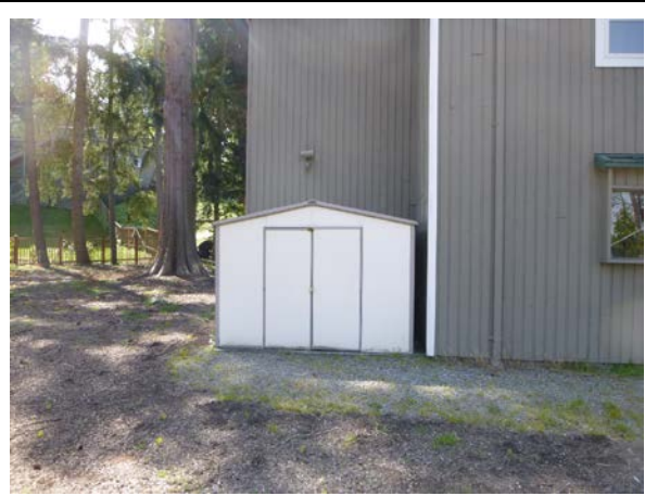
Plate 2. View of the proposed building addition location, looking west.
